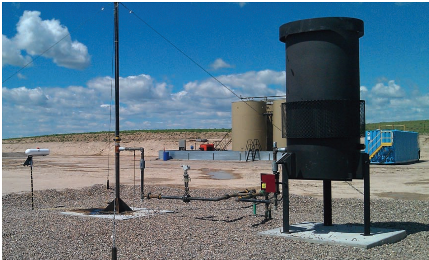
Cimarron's wide range of environmental solutions include Emission Control Devices (ECDs) designed to destroy environmentally harmful emissions created during the energy production process.
